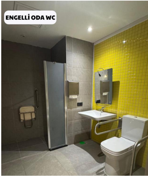
Image 18. Accessible Restrooms in Student Dormitories
